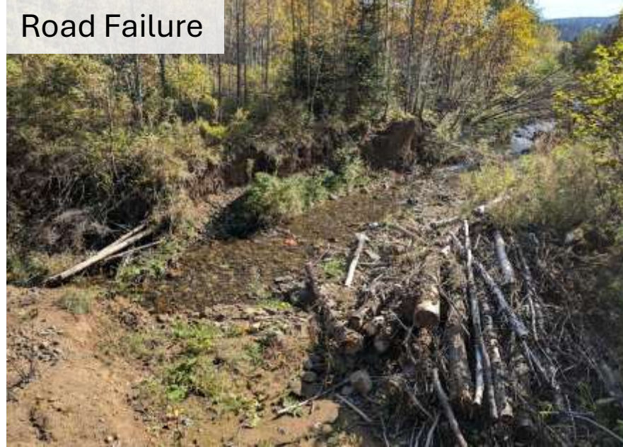
Culvert Scouring & Undersized Culvert
